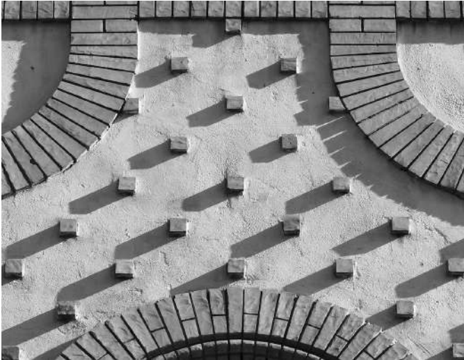
Figure 21. Façade of the neighbouring school-building of the Novi Sad synagogue with brick scoring © Oszkó Ágnes Ivett
