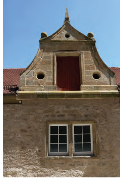
Figure 5. One of the wall dormers with an obelisk, Photo by S. and T. Berger
