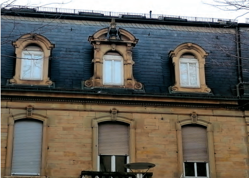
Figure 2. Myliusstraße 8, detail. Photo by S. and T. Berger
