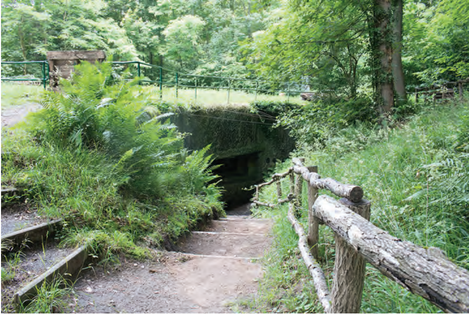
Figure 1. Entrance to one of 17.800 bunkers of the “Westwall” from World War II. Photo by S. and T. Berger
